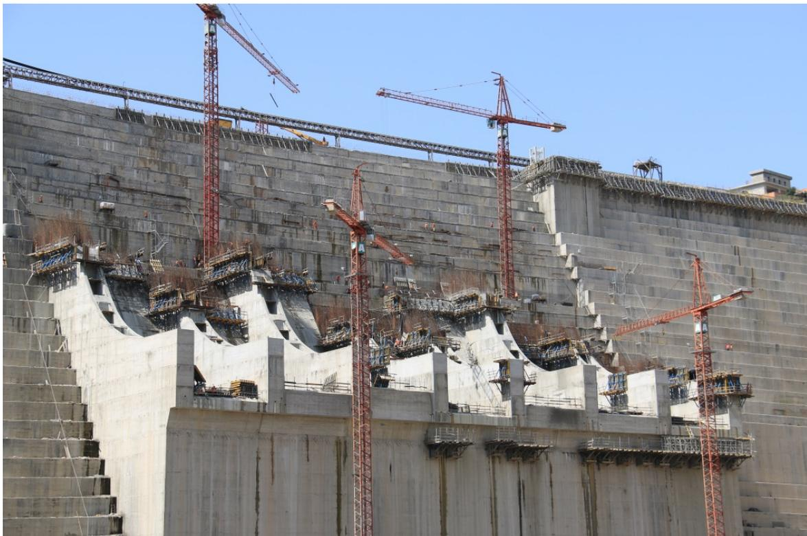
*Fig. 9: Spillway chute under construction*
