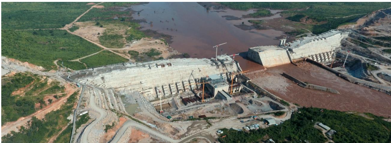
Fig. 1 – View of the GERD project under construction (October 2016)
